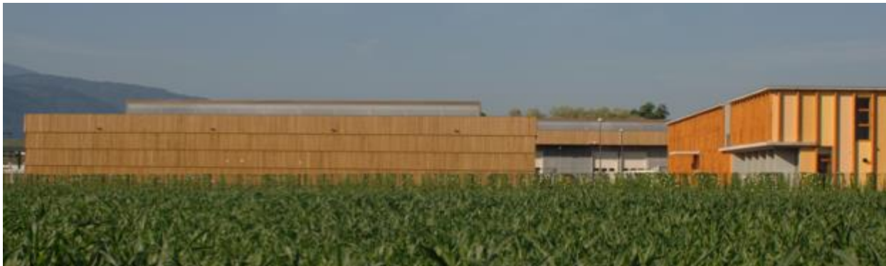
Centre Technique, Crolles (38)
